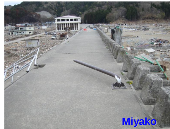
Destruction by wave pressure
